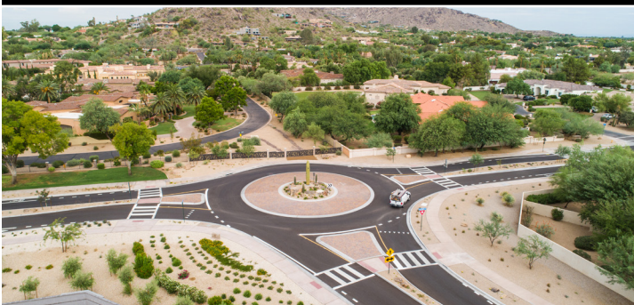
Roadway Improvements to Lincoln, Mockingbird, and Indian Bend / CMAR / Town of Paradise Valley
